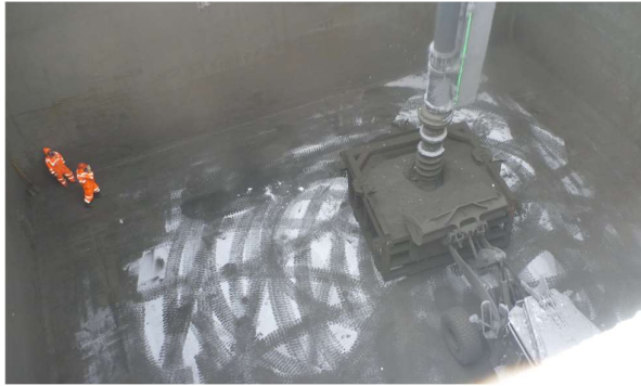
Figure 10 – Nettoyage final de la cale
