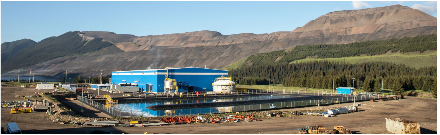
View of the Fording River Operations South Active Water Treatment Facility
