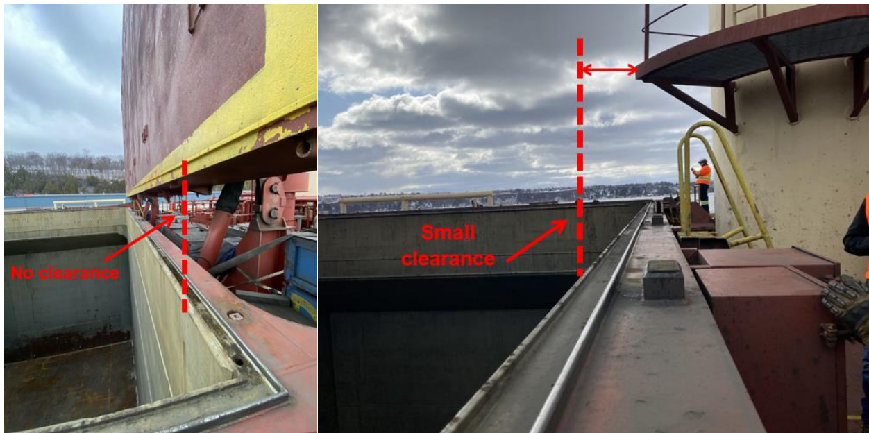
Figure 5-4: Clearance on the Existing Hold Cover and Crane Side
