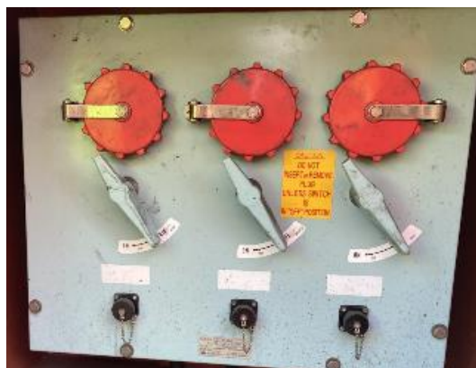
Figure 7-14: 440Vac 60Hz-3p Fused at 30A
