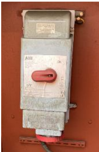
Figure 7-13: 440Vac 60Hz-3p Fused at 60A
